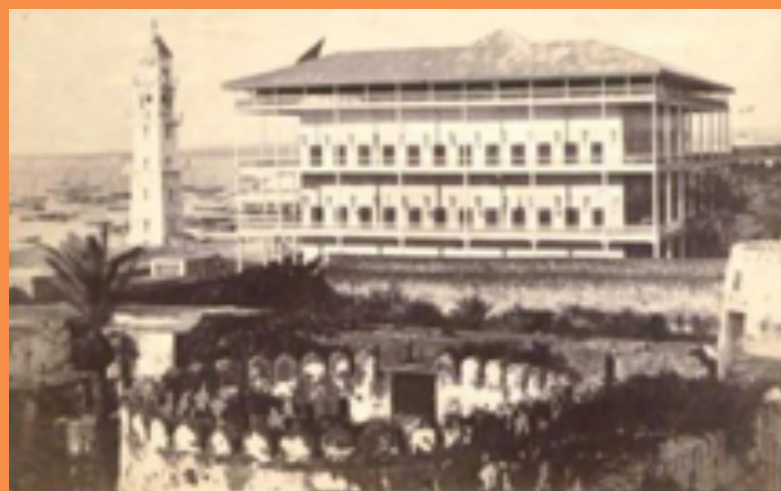
... and after completion
