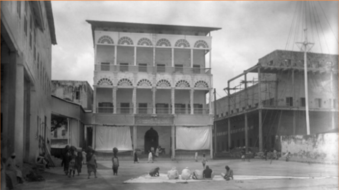
To the right of Beit Al Hukum is the start of construction of Beit Al Ajaib in 1883.
